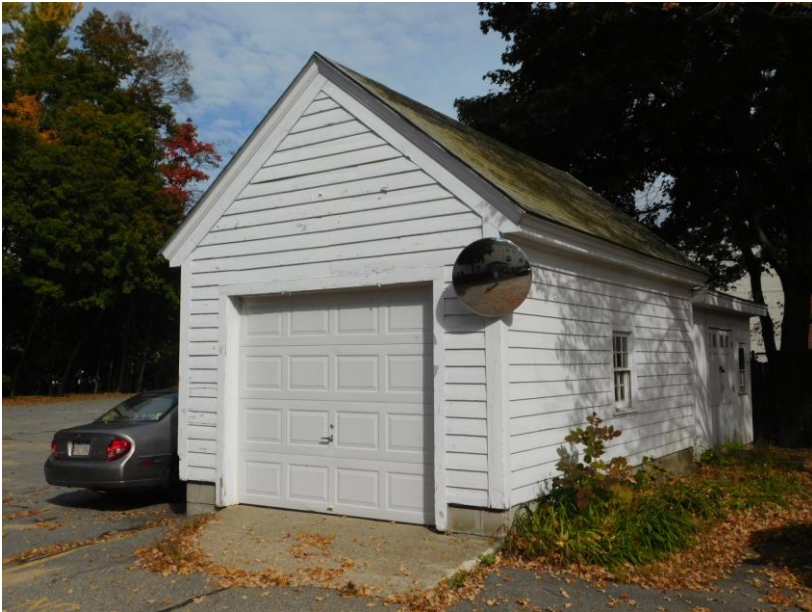
View of garage from SW.
